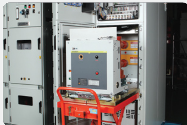
Fig.7 Main switching device & LV compartment
